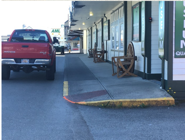
Main Street Non-Compliant Pedestrian Ramps
